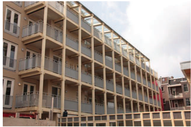
Figure 3: Structural Accoya® (columns, decking and window frames) at FagelCats building, Amsterdam, the Netherlands.
