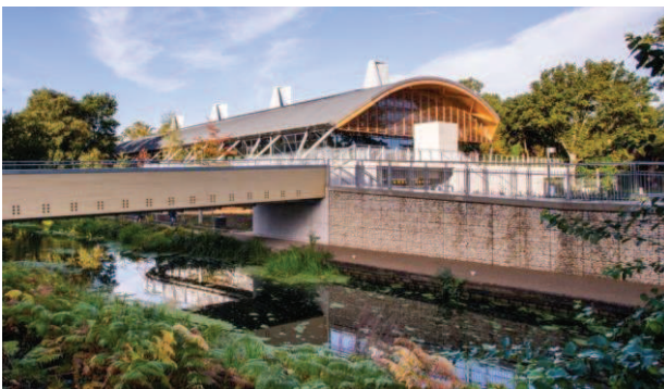
Figure 2: A bridge built at the World Wide Fund for Nature (WWF) headquarters in Woking, Surrey, UK involved 21m 3 of Accoya wood.
