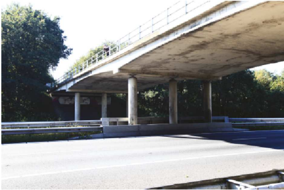
Figure 5. Viaduct de Beek.
