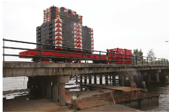
Figure 3. Load application system with steel spreader beam, counterweights, and hydraulic jacks on the Ruytenschildt Bridge.
