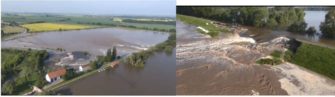
Figure 3.5. Left: overview photo of the inland while the flooding evolves, Right: overview photo of the breach at 10-jun-2013 (Grubert, 2013b; Weichel, 2013)
