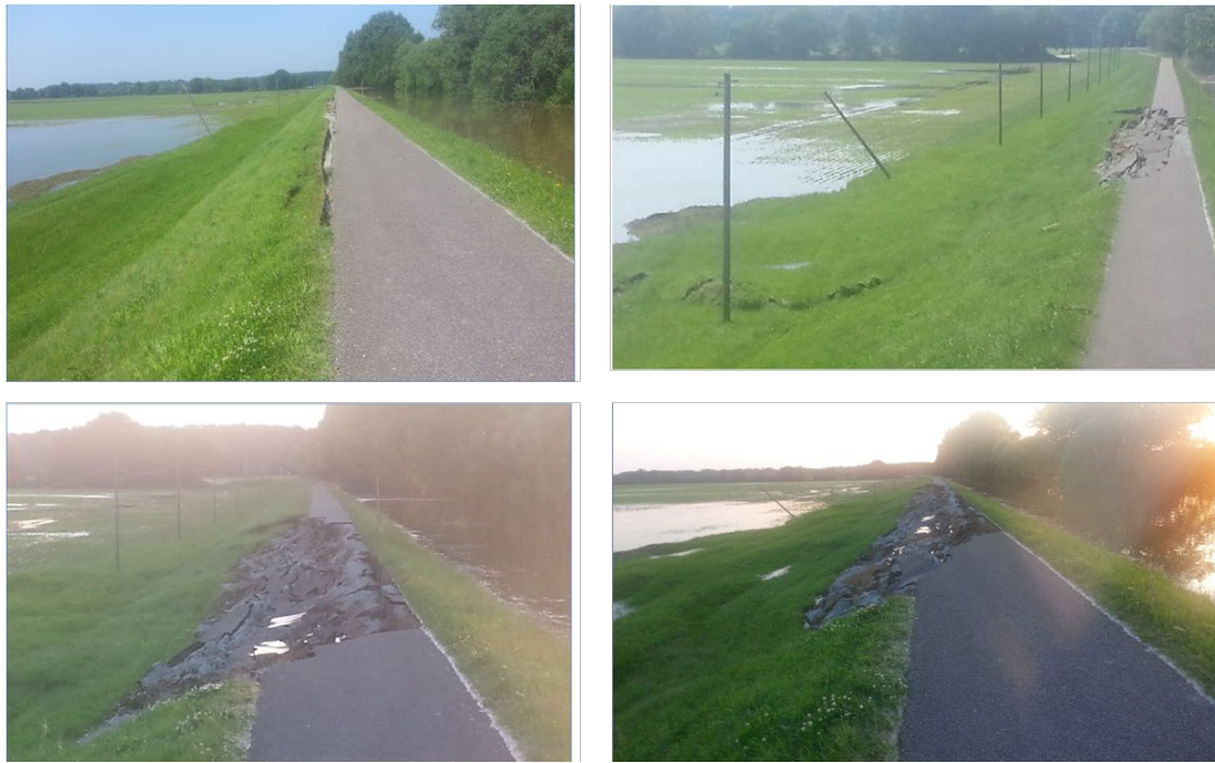
Figure 2.6. Photo series over time (upper left: 08.06.2013-10:37, initial break at the edge of the slope, upper right: 08.06.2013-14:10, horizontal shifts, bulge of the toe, lower left: 08.06.2013-20:51 continuing failure, lower right, 08.06.2013-20:55, continuing failure) with the visual predictors (Grubert, 2013a). The riverside of the levee is on the right for all photos.
