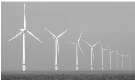
Figure 1. Egmond aan Zee Offshore Wind Farm (Netherlands).
