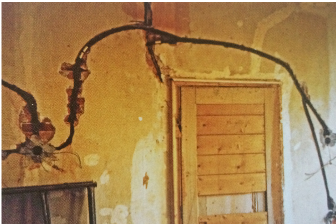
Figure 29: Not reversible cabling (Source: Nusselder)
