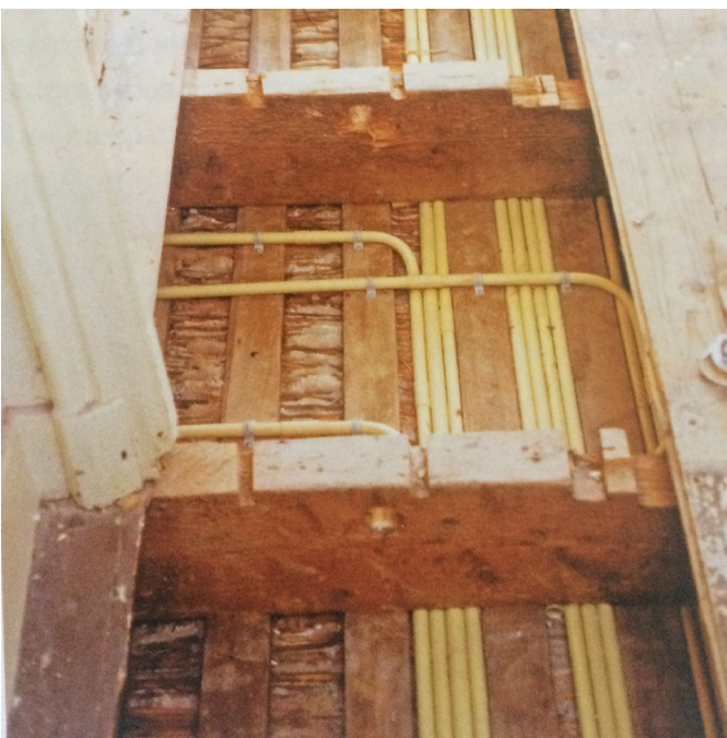
Figure 30: Reversible cabling (Source: Nusselder)
