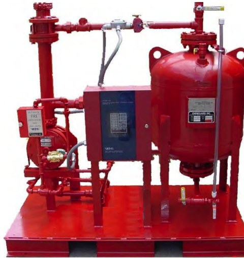
Figure 10-4: Example of a Foam Mixing System [24]
