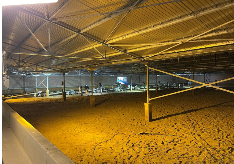
Figure 4: Scraping of a slow sand filter (scraped bed)
