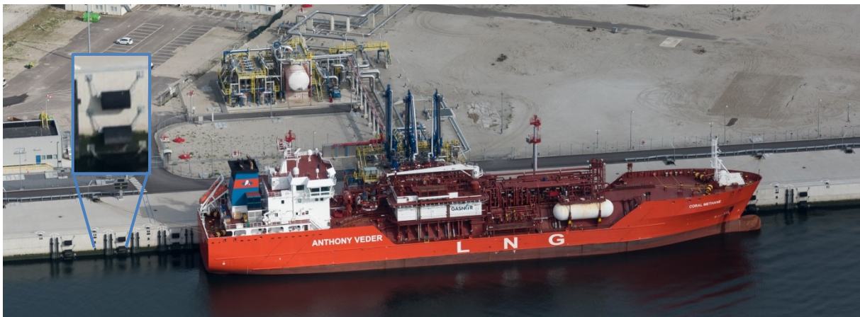
Figure 8: Gate Jetty 3, the Small Scale facility (Photo Paul Martens).
