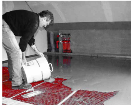
2 installation of the capillary tube mats directly in the Levelling Compound (Clina, 2016)
