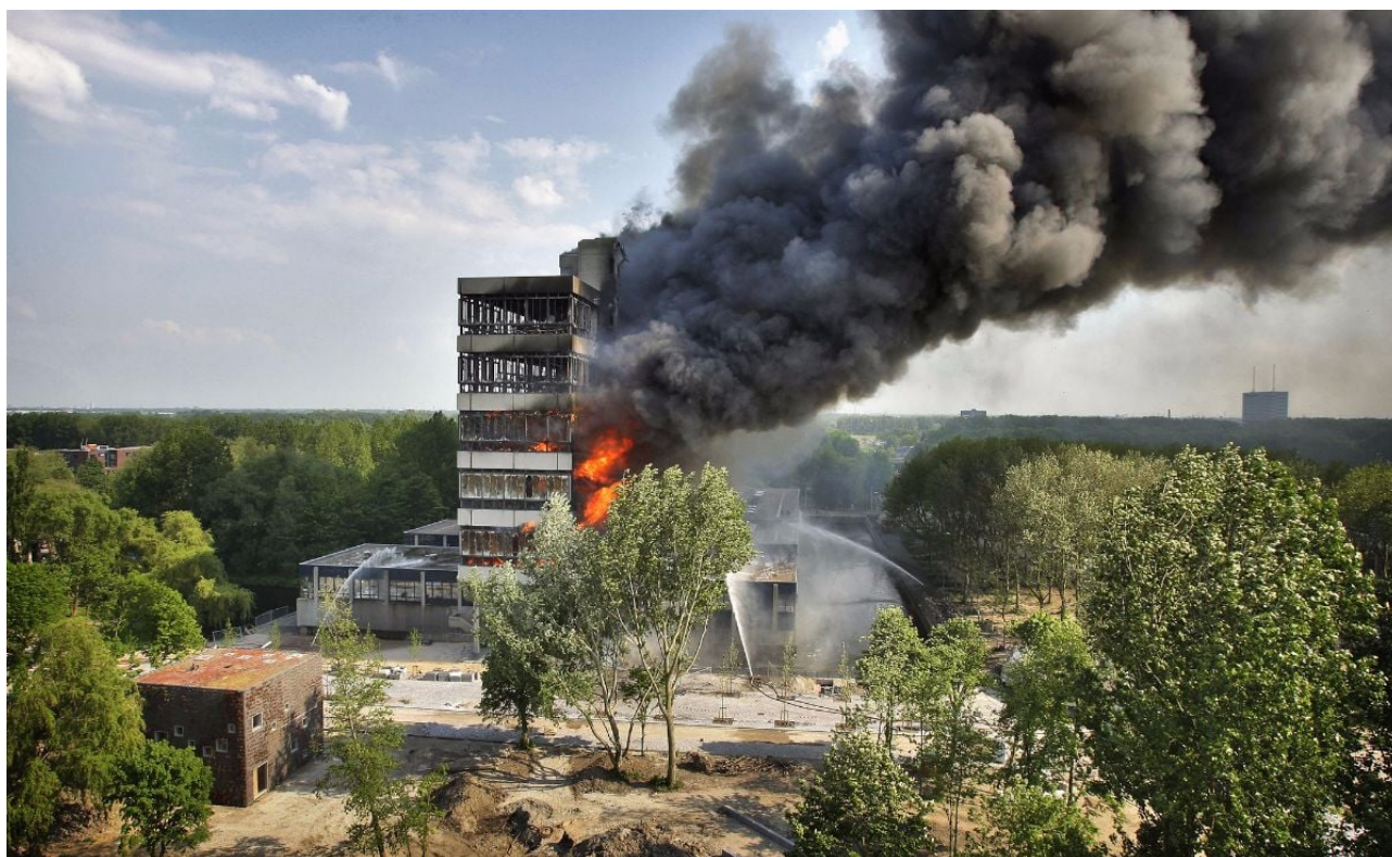
Figure 2.1: Fire at the TU Delft Faculty of Architecture on May 13, 2008 [97]
