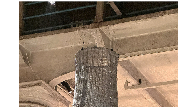
Fig. 10. Top: Closeup of the funnel support showing the ring cross-section with (a) the suspension cable, (b) threaded chain, (c) stainless steel compression ring, and (d) integrated channel in the knit. Bottom: Final funnel support.
