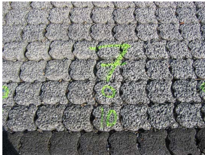
Foto 6-2 Hydroblocks in Bath. Hier proef 7 steen 10.
