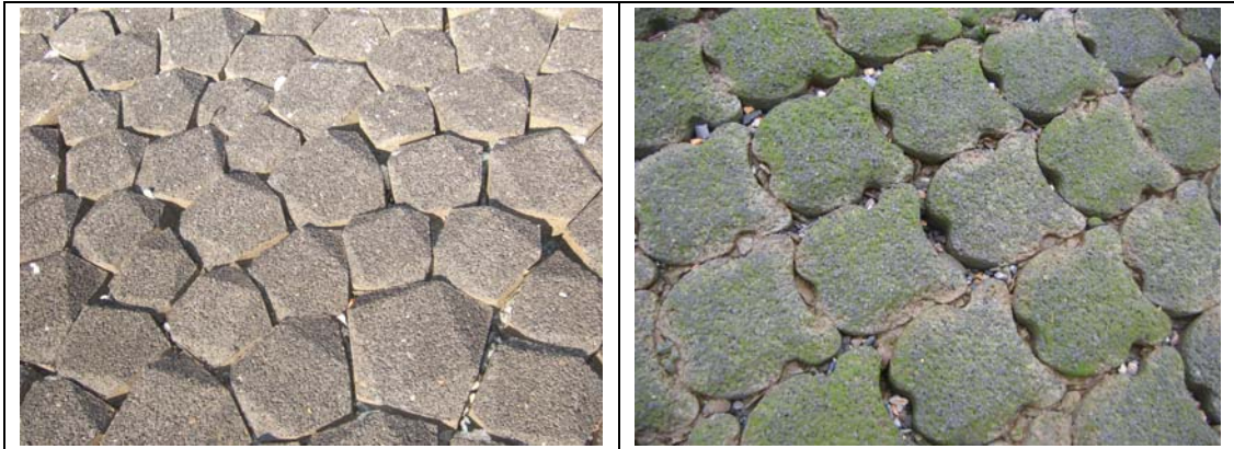
Foto 2-2 en 2-3 Basalton (Sluis) – Hydroblock (Bath)
