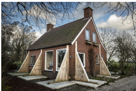
Figure 1.4: Typical Dutch detached house with OOP retrofitting.
