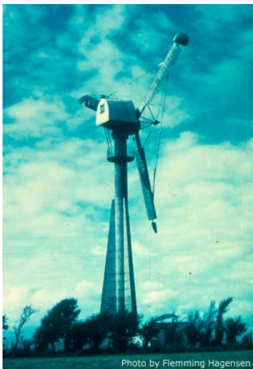
Figure 2.12: The Gedser turbine. The mother of modern low speed 3 bladed upwind wind energy converters.
