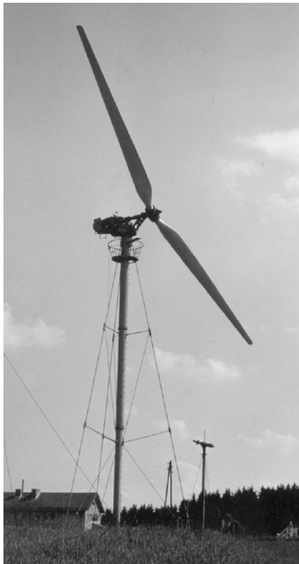
Figure 2.10: The W34 wind turbine (rotor dia. 34m, rated power, 100kW), Stötten, Germany, 1959 [9].
