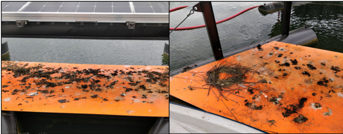
Figure 4.7: The two heavily soiled reflectors of the Retractable System.
