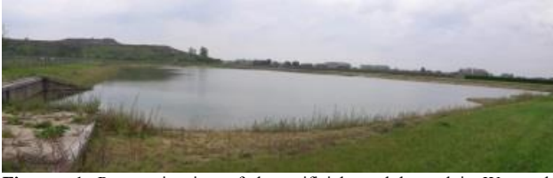
Figure 1. Panoramic view of the artificial pond located in Weurt, the Netherlands (51.8514 ° N, 5.7950 ° E). The pond is developed as a water retention basin. The pond has a rectangular shape, not perfectly aligned with the South. The longer side of the pond is 42° deviated towards the West (222°).
