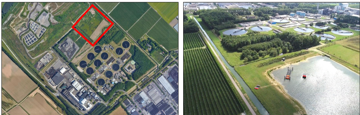
Figure 1.5: The picture on the left shows the location of the floating PV pilot system in Weurt, indicated by the red square (Adapted from [22]). The picture on the right shows a bird's-eye view of the pilot system.
