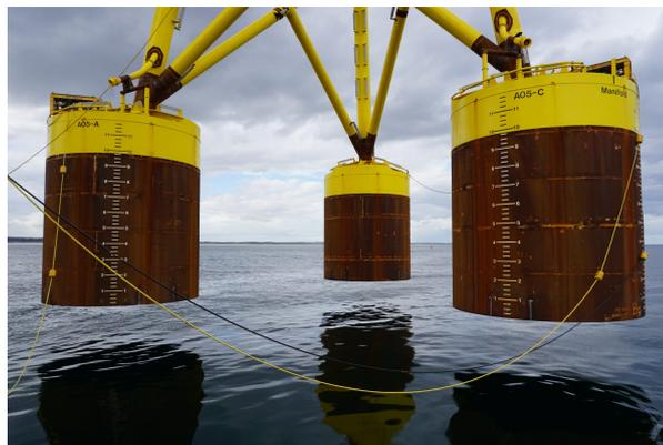
Figure A.10: Suction Pile by SPT Offshore
