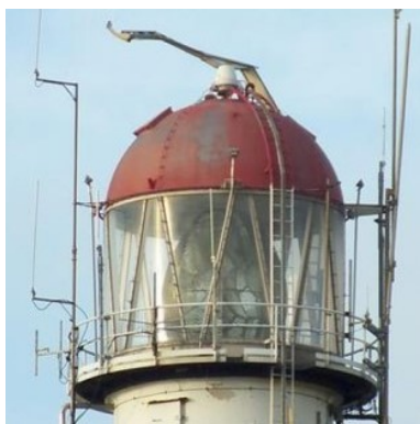
(a) Destroyed radar system at the lighthouse
