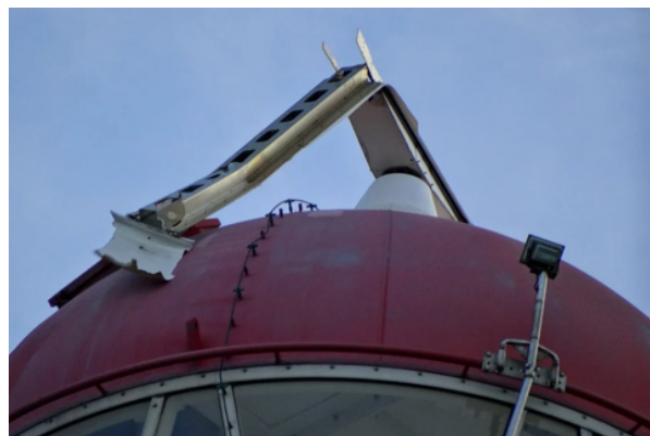
Figure 5.5: Failure of the radome in the Lange Jaap incident
