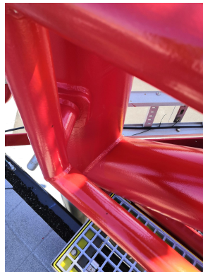
(a) Welding between members in the mast
