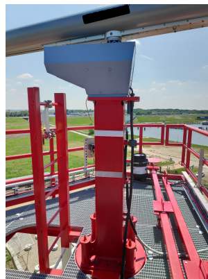
Figure 5.1: Nautical radar system on the mast in Stellendam
