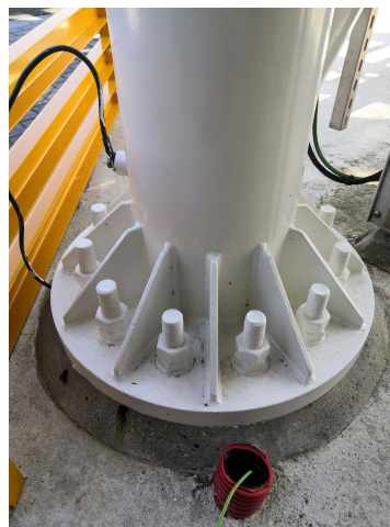
Figure 4.7: Base of the column
