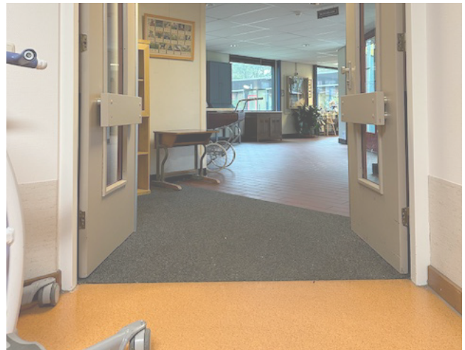
Image 40: Contrast between flooring (Own work, 2024)
