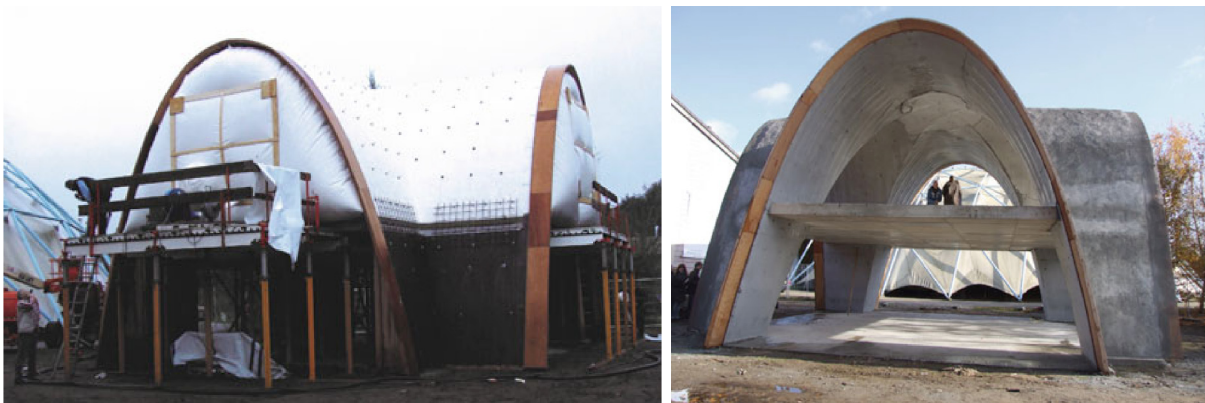
Figure 68: Prototype cross vault by R. van Hove Left: inflatable mould, Right: concrete shell. Source: Pronk, 2021.
