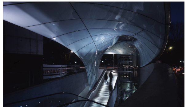
Figure 60: Up: Steel-rod mould of the Nordkettenbahn. Source: Rietbergen, 2008. Down: Nordkettenbahn by Zaha Hadid. Source: www.zaha-hadid.com
