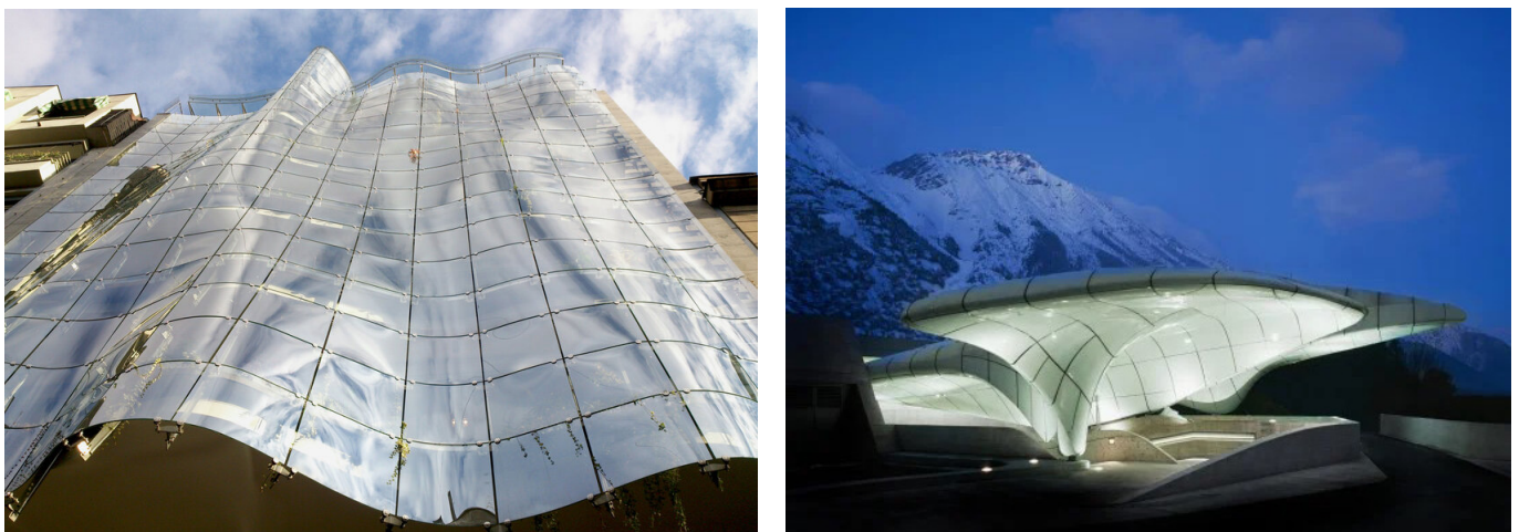
Figure 21: Left: Infinity residential building. Source: Alfirevic, 2013. Right: Nordkettenbahn station. Source: www.baunetzwissen.de .
