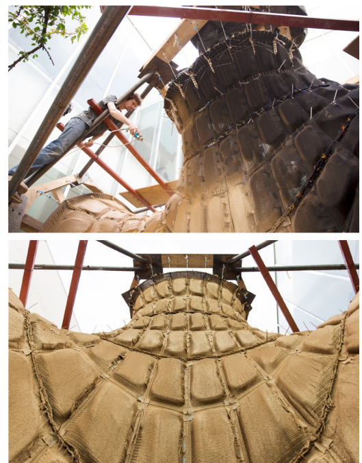
Figure 92: Up and Middle: Cement coating application on knitCrete bridge prototype. Down: Mortar application on top of coating, knitCrete bridge prototype. Source: Popescu,2019.
