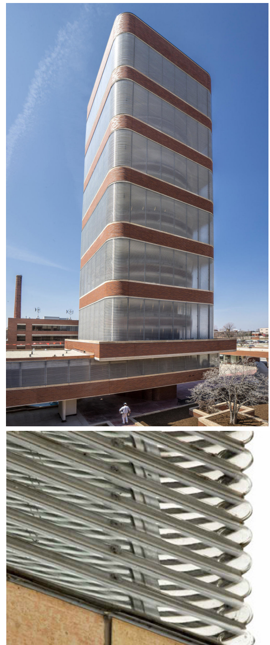
Figure 44: Johnson Research Tower extruded glass facade. Source: up: www.elevatorscenestudio.com . down: Oikonomopoulou, 2019.
