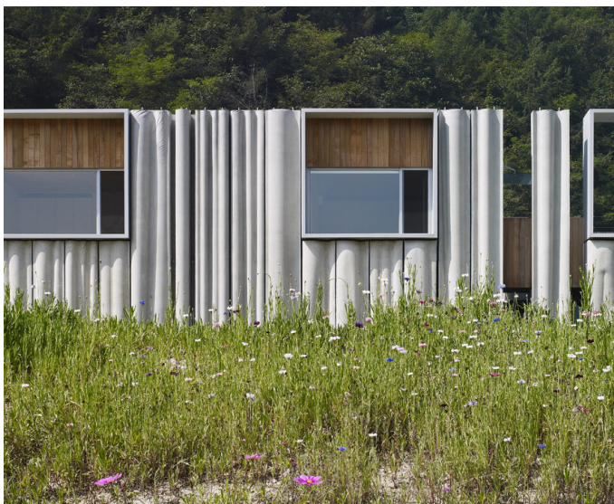
Figure 7: Hanil Company Visitors Center façade: prefab concrete panels formed with open through fabric moulds. Source: www.archdaily.com
