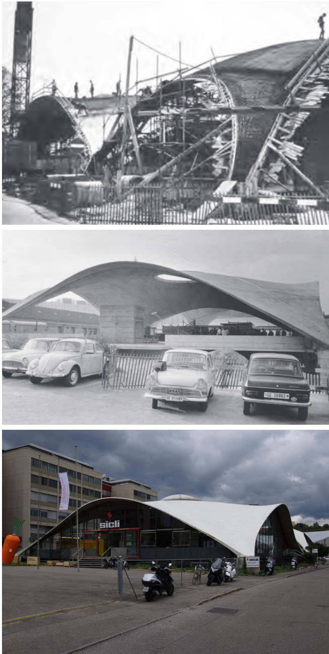
Figure 76: Up: Sicli roof with formwork and Middle: Sicli shell. Source: Delemontey, 2019. Down: The Sicli pavilion. Source: www.structurae.net.
