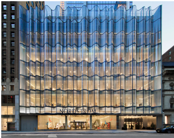
Figure 1: Corrugated glass facade of the Nordstrom flagship store in NYC. Source: www.press.nordstrom.com
