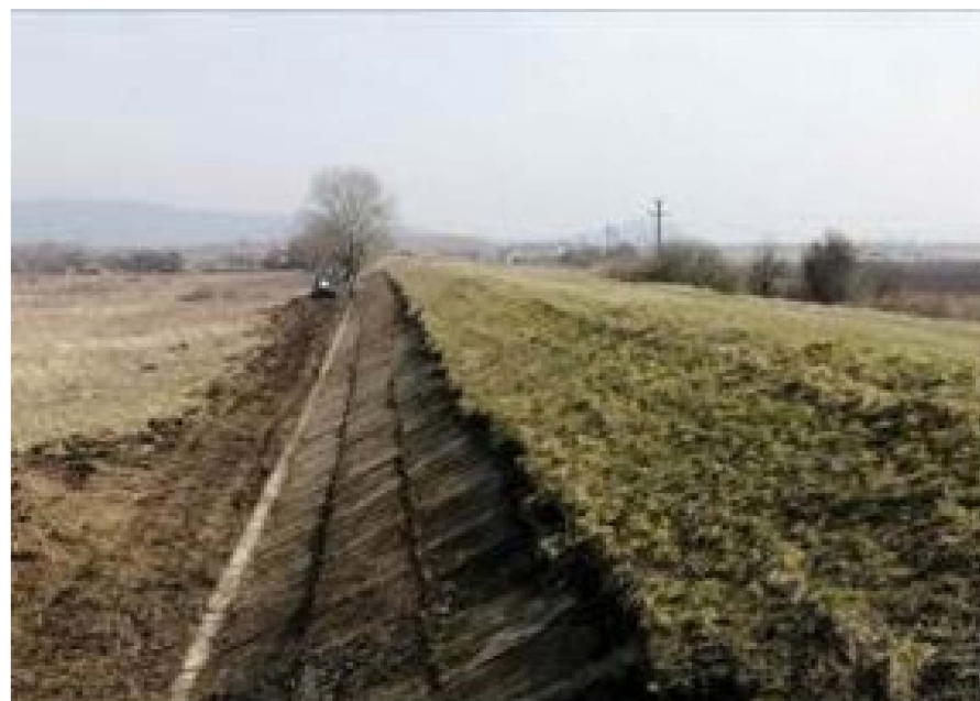
Figure 8. View of Deva flood protection levee.
