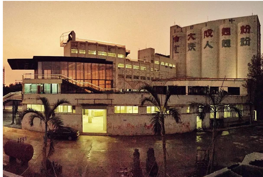
Dacheng Wheat Flour Factory, the first factory established by foreign investment In 1980s, Shekou, Shenzhen
