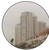
:Apartment blocks almost finished; most units have sold.
