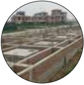
Foundations of An Khanh An Thuong residential neighborhood.
