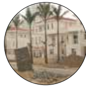
:Villas almost completed; 100% have owners.
