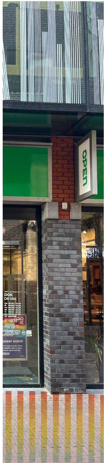
2. Facade consists of masonry and glass windows, similar stone pavement(own image)
