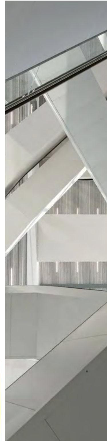
4. Escalators, stainless steel stairs with glass railings, acoustic ceiling panels (own image)
