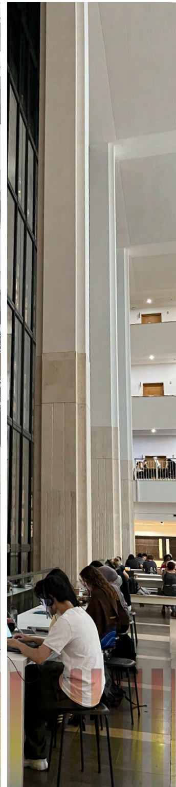
7. Natural stone flooring, plaster and glass walls, perforated acoustic ceiling panels (own image)
