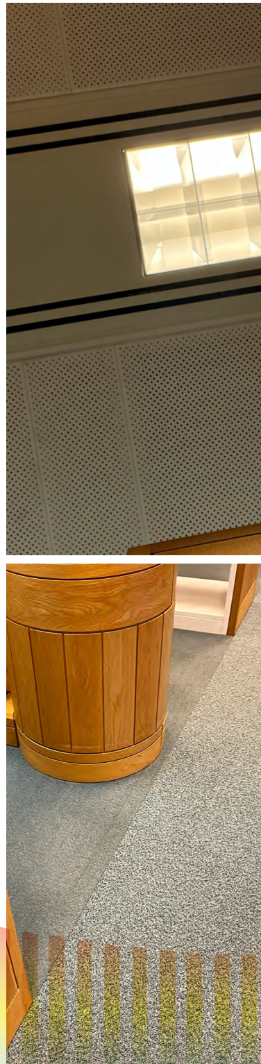
4. Carpet flooring, wooden furniture and perforated acoustic ceiling panels (own image)
