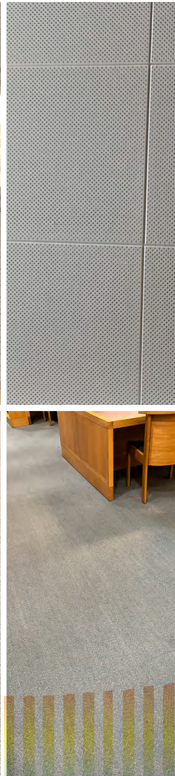
5. Carpet flooring, wooden furniture and perforated acoustic ceiling panels (own image)
