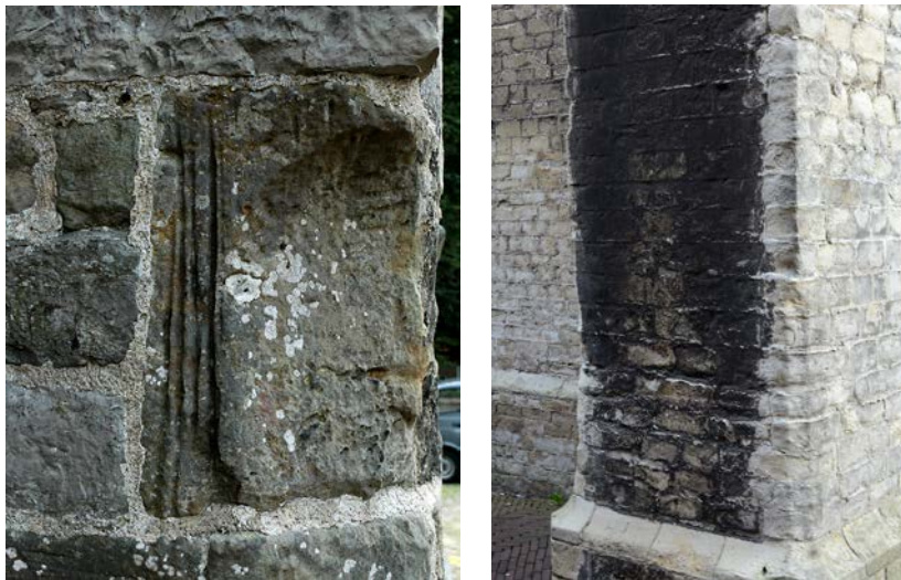
Figure 2 Left: Highly valued man-made traces at St. Bavo Church Aardenburg, right: black crust due to weathering at Old Church Delft (photos; W.J. Quist).
