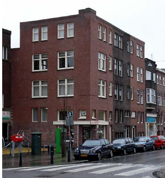
Figure 1 Although technically not necessary, visible traces of ageing are often removed, i.e. when cleaning brickwork facades (photo: W.J. Quist).
