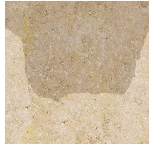
Wet concrete Surface
