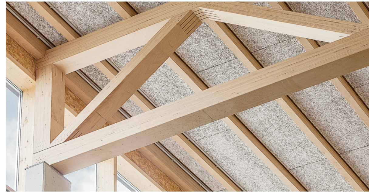
BauBuche truss with BSB connections, i+R Holzbau
