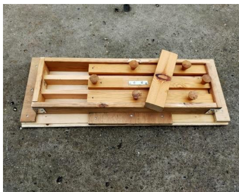
Fig. 13 - Shrink box formwork
