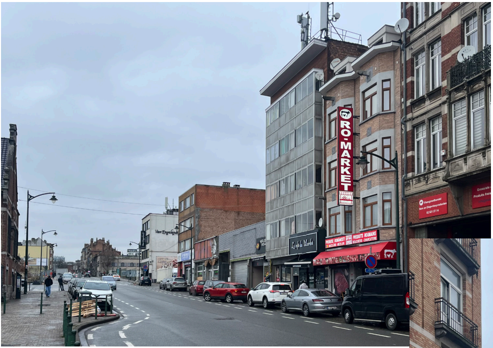
View of the site's facade on Rue Ropsy Chaudron
