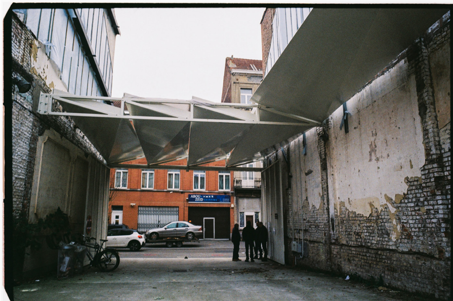
Similar passage conditions in Heyvaert
