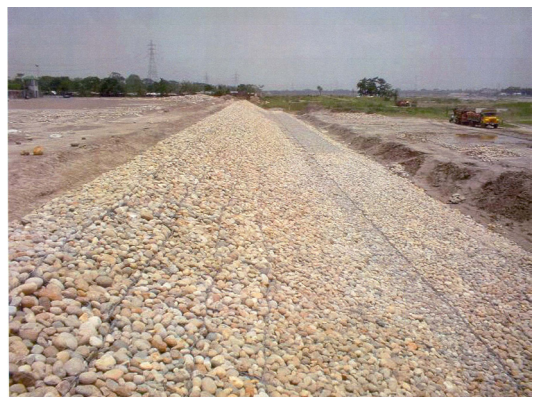
Figure FS2.2: Gabion mattress on a slope of a future river bank
