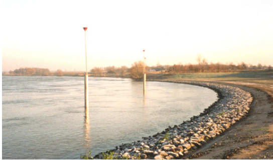
Figure FS4.1: Rockfill river bank protection
