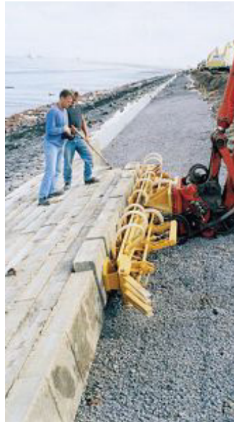
Figure FS5.2: Concrete tiles placed by special equipment
