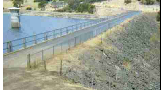
Figure FS4.2: Rockfill spillway
