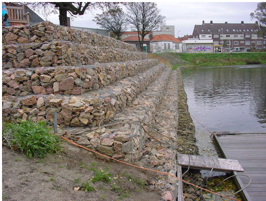
Figure FS2.1: 'Stepped' gabion in urban river bank
