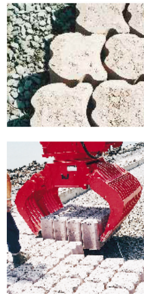
Figure F5.3: The placement of special concrete blocks
