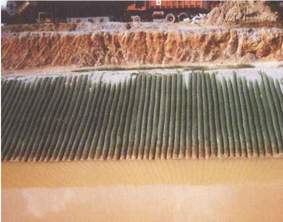
Figure FS6.1: Application of a cellular geo-mattress on the outer slope of an embankment
