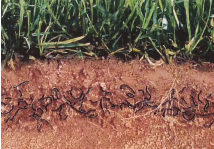
Figure FS1.1: Cross section of a reinforced grass revetment
