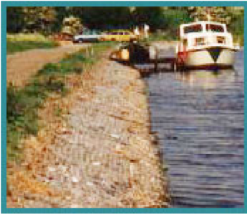
Figure FS2.3: Gabion riverbank protection just after construction
