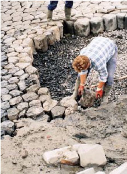
Figure FS5.1: Craftsmanship; basalt columns placed by hand
