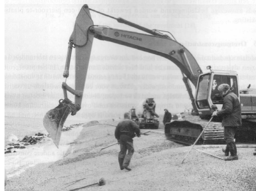
Figure FS9.2: Placing concrete with a hydraulic crane
