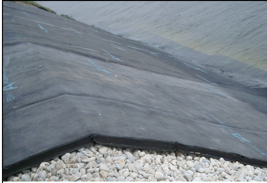
Figure FS8.1: Preparation for asphalt works
