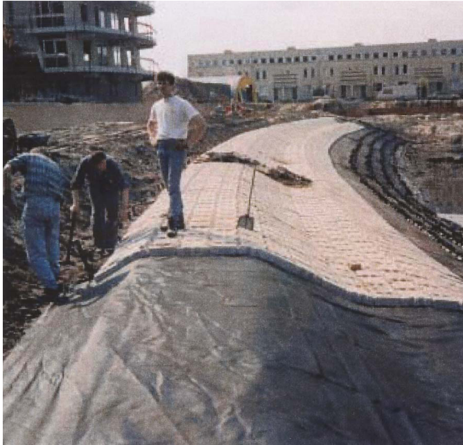
Figure FS3.1: installation of an open concrete block mattress
