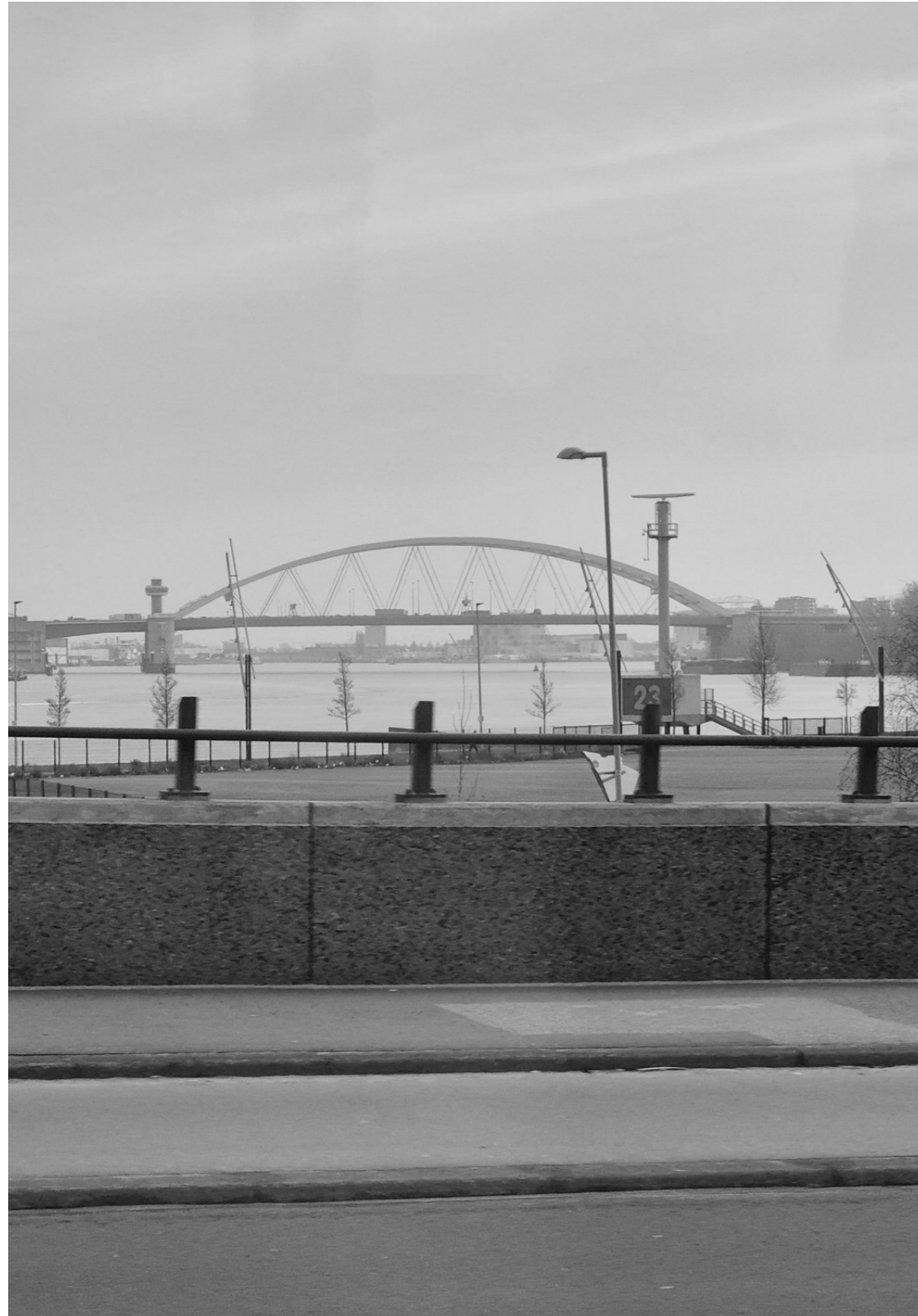
The Brienoord Bridge (Image made by author)
