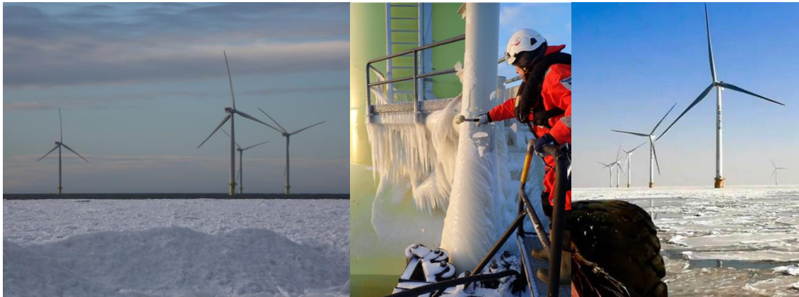
Figure 1. Left: Fast ice in the vicinity of the Tahkluoto wind farm (picture courtesy of Cody Owen). Center: Icing on a boat landing and ladder. Right: broken ice near turbine foundations in the Bohai Sea (picture courtesy of prof. Qu Yan).
