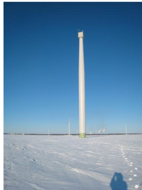
Figure 3. 3 MW OWEC test foundation in land-fast ice in 2010 (Picture source: Määttänen, 2010).
