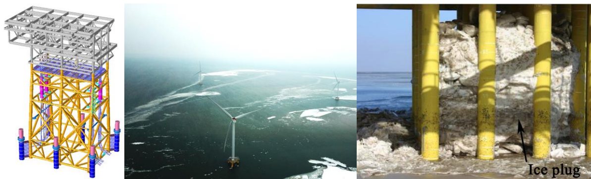
Figure 7. Left: An example concept of a substation jacket with nine members of different size penetrating the waterline (illustration courtesy of Kasiphon Kurojjanawong). Center: Jacket support structures in ice at the Nissum Bredning wind farm in Denmark. Right: Ice plug inside casing pipes in 2021 in the Bohai Sea (picture from Wang and Zhang, 2023, CC BY 4.0 DEED).
