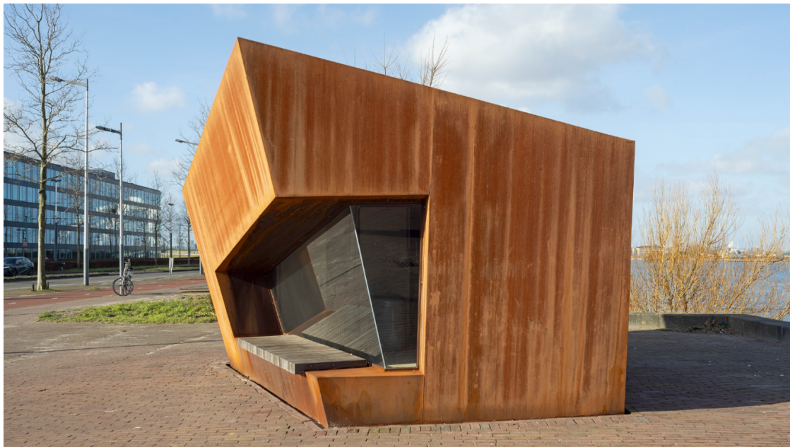
Figure 2.15: A Heat Transfer Station in Amsterdam [56]
