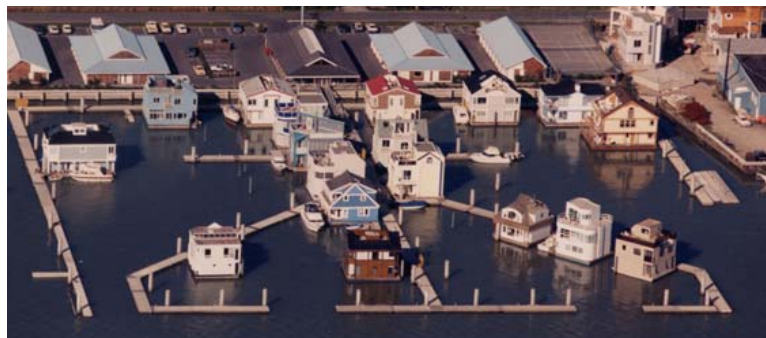
Figure 2: Floating quarter in construction (www.floatingstructures.com)
