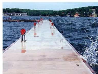
Figure 13: Floating Breakwater, IMF
