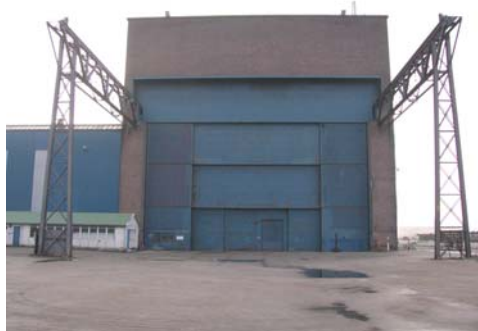
Figure 29: Large assembly hall at Heijplaat
