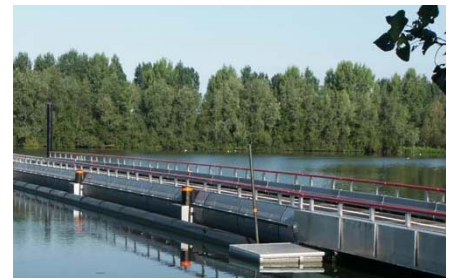
Figure 11: Floating Road, Hedel
