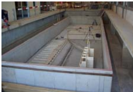
Figure 20: Concrete Casco [Arkenbouw Post]
