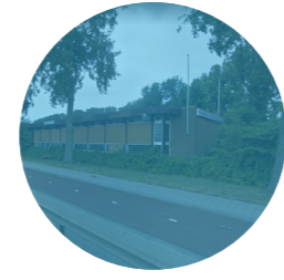
Seamens Centre (vacant)
