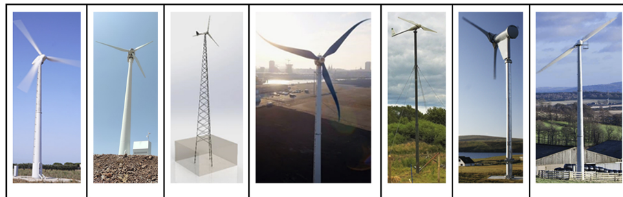
Figure 12. Common HAWT archetypes found on the current DWT market. From left to right: upwind, active pitch and yaw (photo credit: Tozzi Nord); upwind, stall-controlled and active yaw (photo credit: Eunice); upwind, stall-controlled and tailed passive yaw (photo credit: NREL pix 49511); downwind, stall-controlled and passive yaw (photo credit: Eocycle – formerly XANT); upwind, tailed passive yaw, furling (photo credit: Bornay); downwind, pitch- or pitch-coning-controlled, passive yaw (photo credit: SD Wind, formerly Proven); downwind, stall-controlled, passive yaw and teeter (photo credit: Ryse Energy, formerly Gaia).
