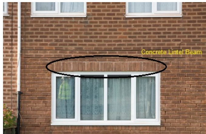
Fig. 3.15.: AS BUILT CONFIGURATION OF LINTEL BEAMS
