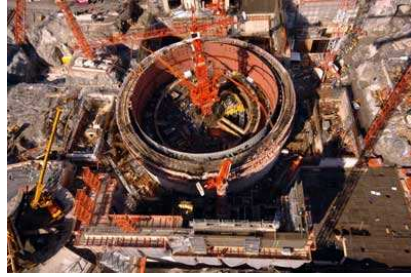
Figure 1.1: The Olkiluoto nuclear power plant under construction
