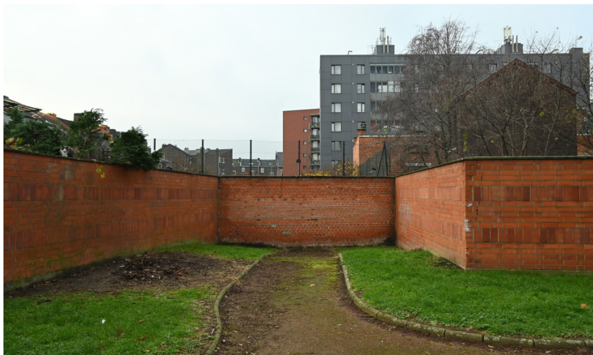
Existing boundary wall
