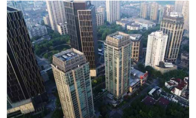
Fig. 1.13 | Shanghai high-rise center
