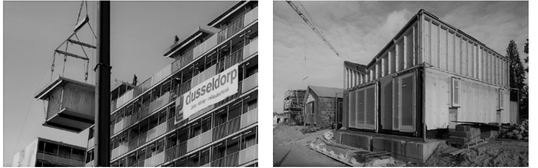
Fig. 6.11 | Circular use modules from common buildings
