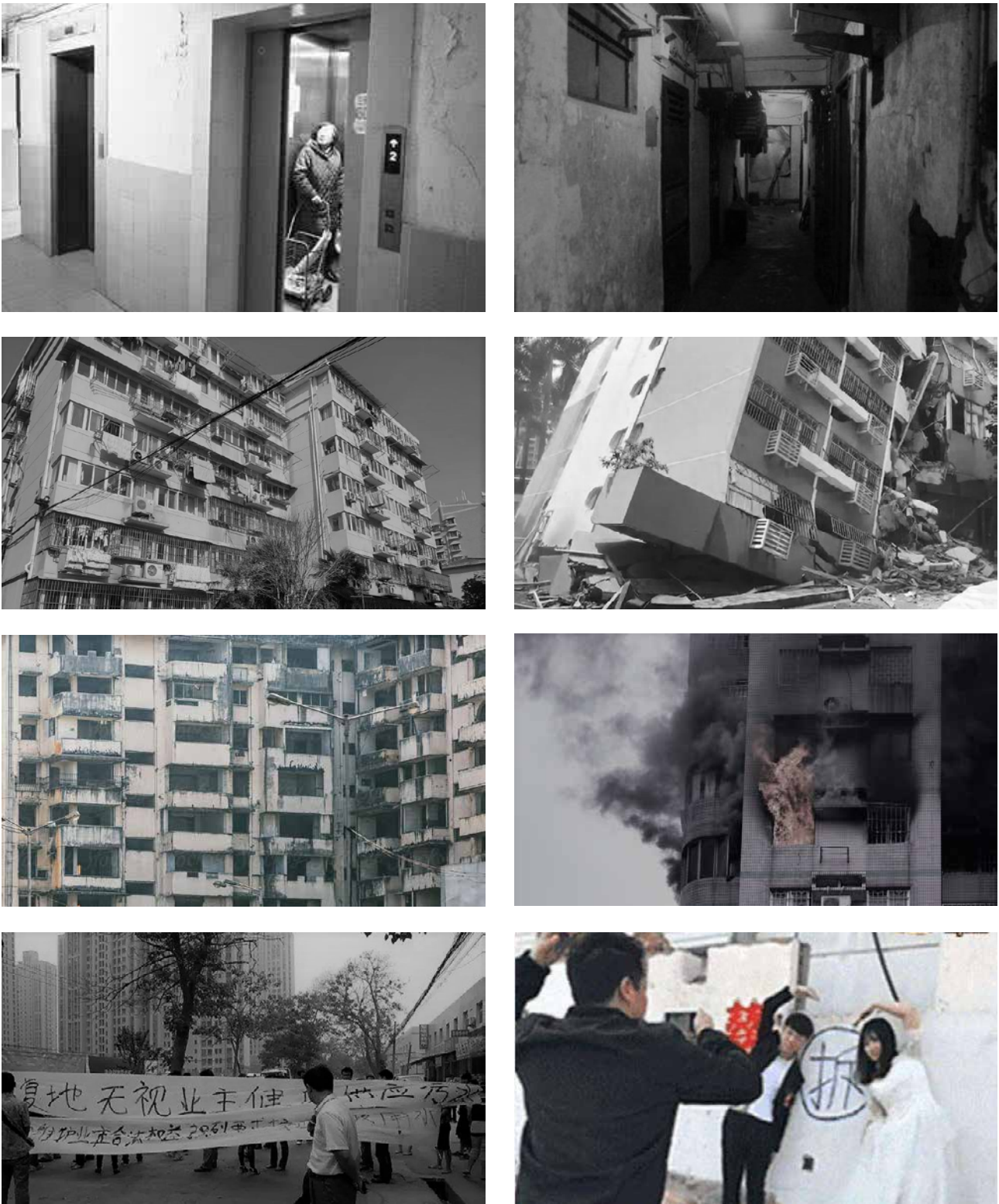
Fig. 1.32| Photos of problems of New Workers' Estates
