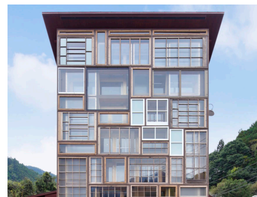
application of remanufactured window frames Kamikatz Public House, © Hiroshi Nakamura & NAP
