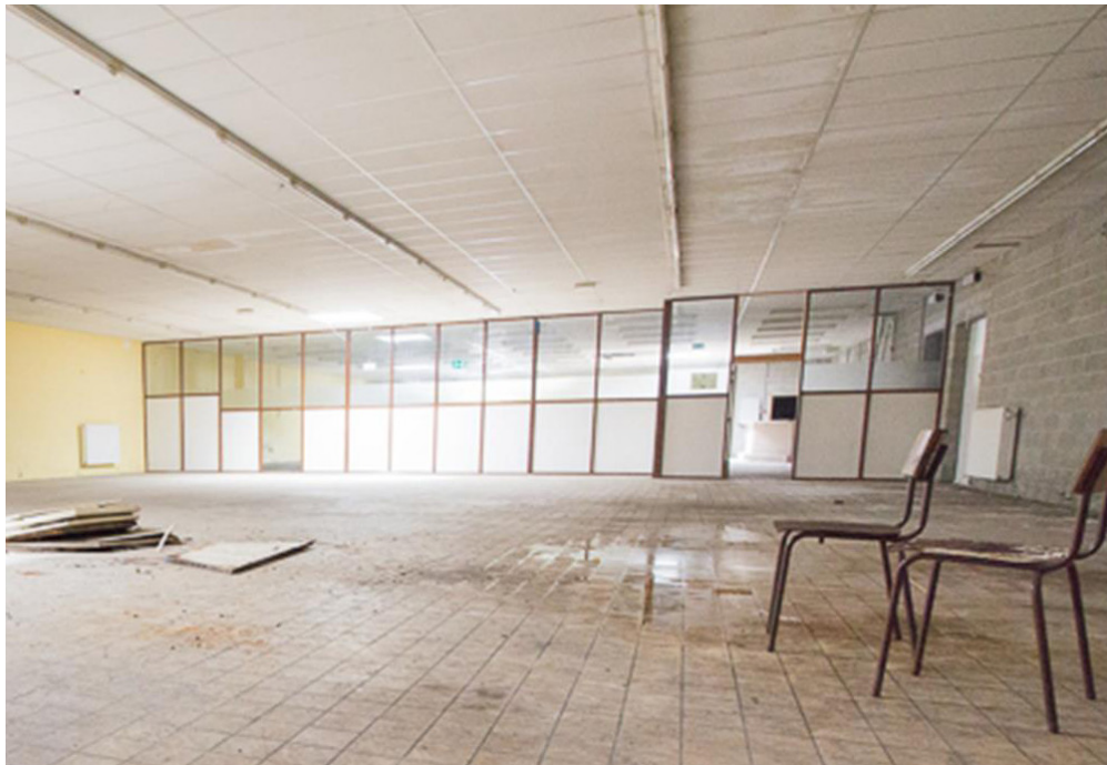
suspended ceiling panel, floor tiles, concrete masonry room divider, radiator, fixture (picture courtesy of realo.be)
