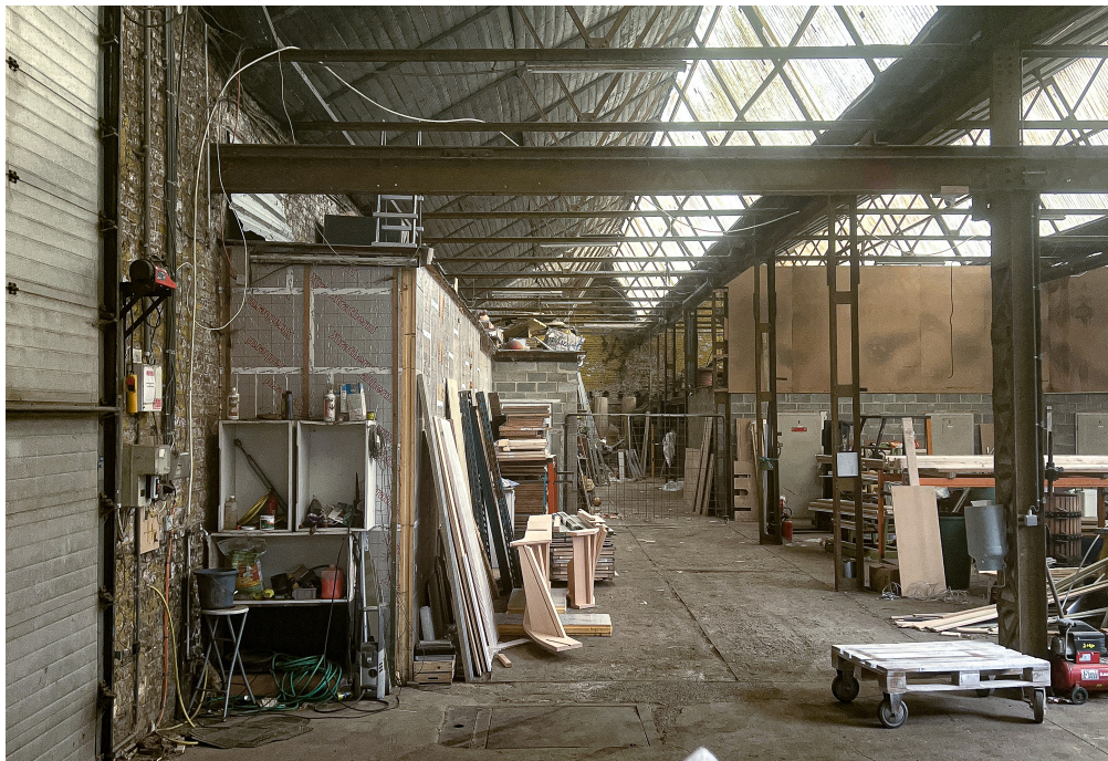
brick masonry, roller door, belgian truss, column, roof decking (picture by Simon van Soolingen)
