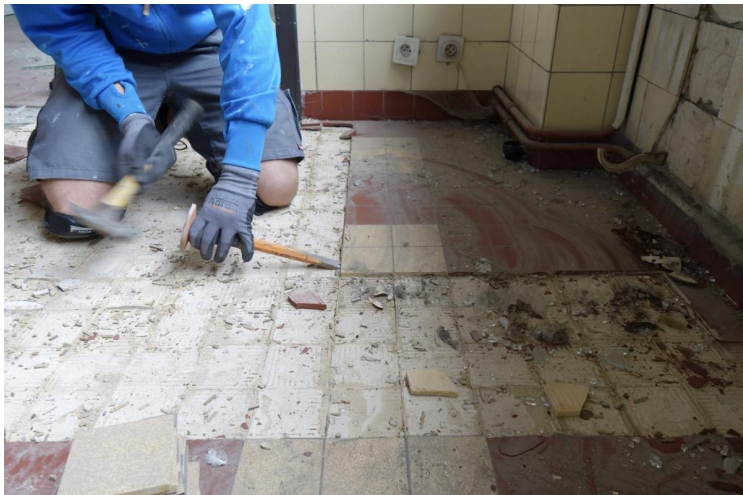
removal of reuseable ceramic tiles © RotorDC
