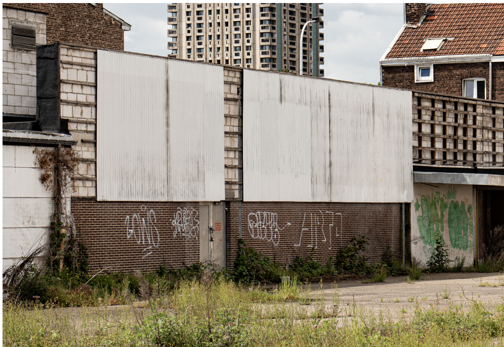
corrugated sheeting, brick work, door, timber framing, concrete masonry (picture by author)
