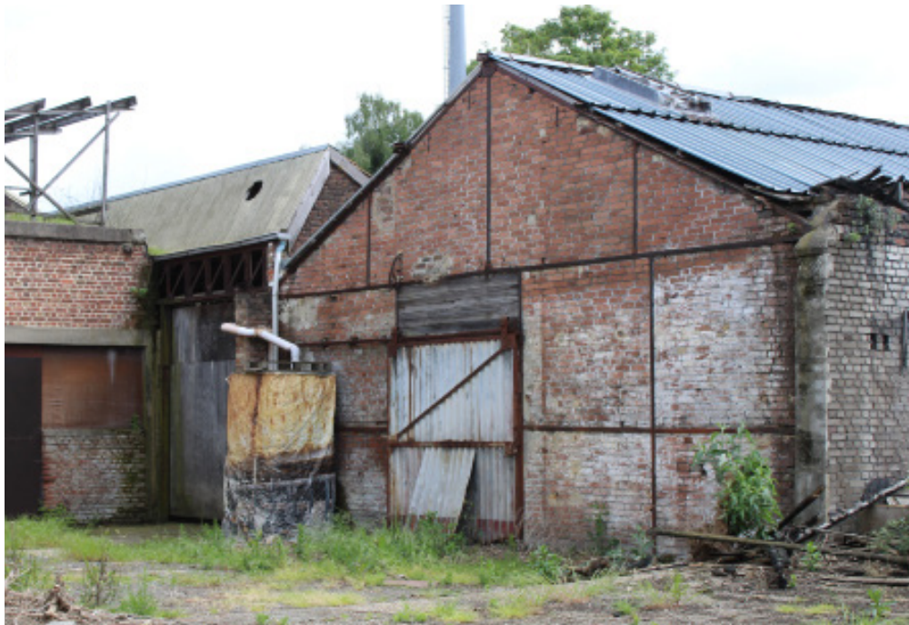
brick masonry, corrugated sheeting, sliding door, straight truss (picture by Wiktoria Paszek)
