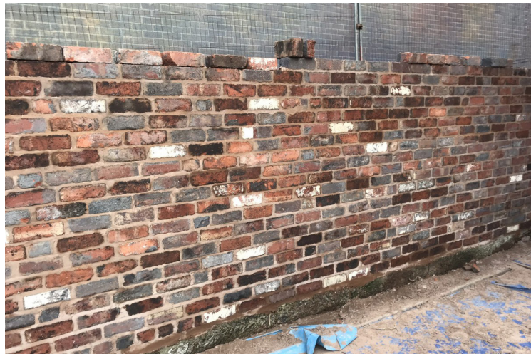
reuse of reclaimed bricks © SalvoWEB
