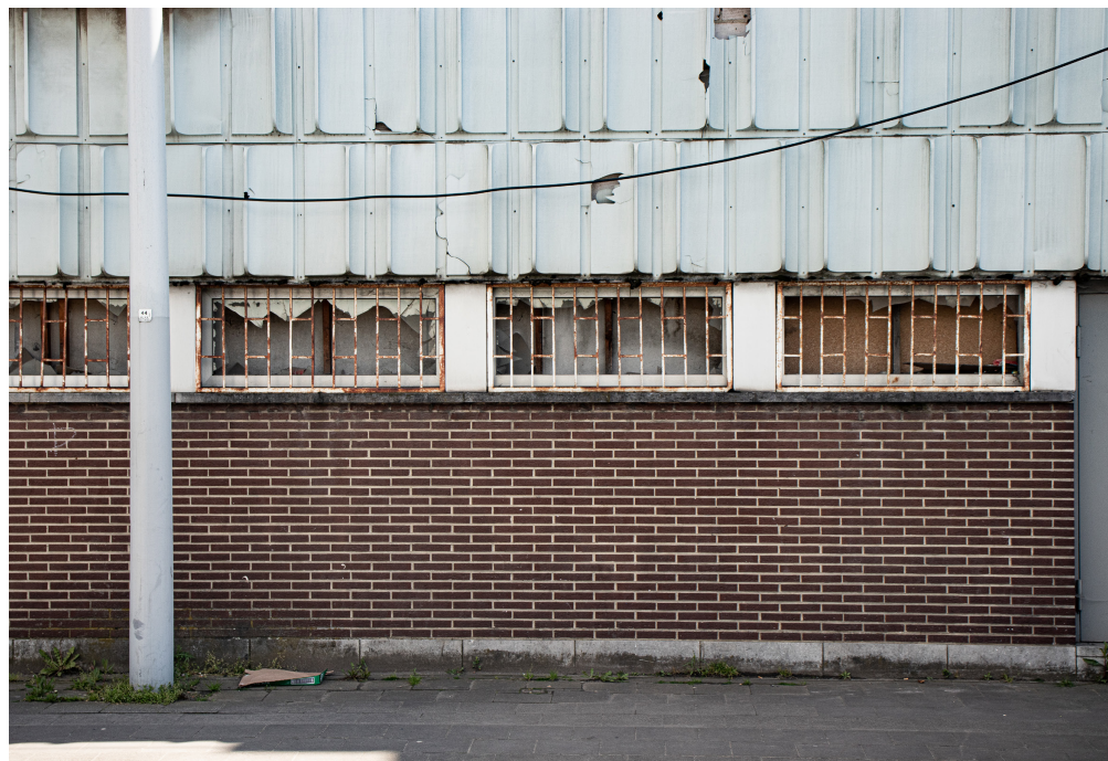
brick masonry, window grill, window frame, facade panel (picture by author)
