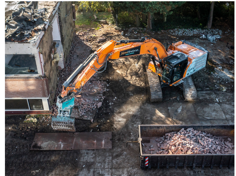
seperating bricks during demolishment © New Horizon
