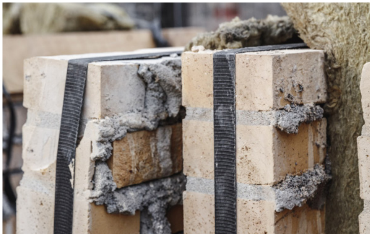
storing cut out brick panels © Lendager
