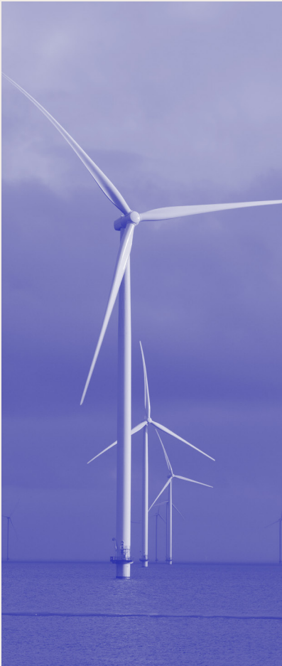
Figure 3.6: Wind farm Fryslan windturbines
