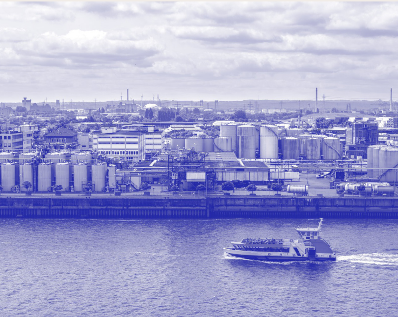
Figure A.5: Hydrogen infrastructure Source: Freepik
