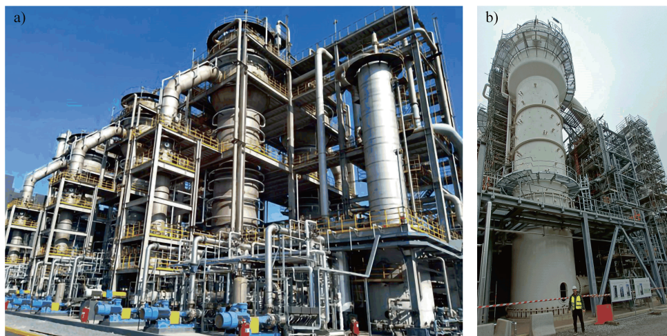
Figure 1.2: Photographs of industrial-scale syngas fermentation plants, depicting LanzaTech's external-loop gas-lift reactors. a) Shougang-LanzaTech plant near Beijing, China 2 , b) Steelanol plant near Ghent, Belgium, the author is visible for scale.
