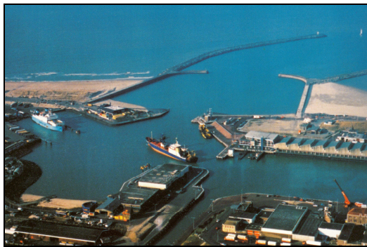
Figure 12.7 Port breakwaters (Misawa, Japan and Scheveningen, The Netherlands)
