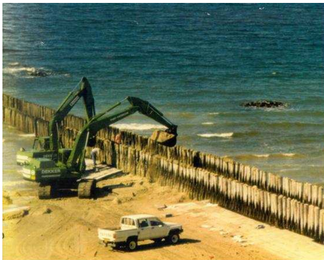
Figure 12.10 Row of piles
