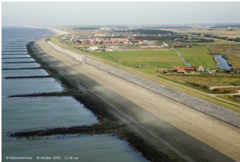
Figure 12.25 Additional sheet piling (Hardly visible at crest of dike.)
