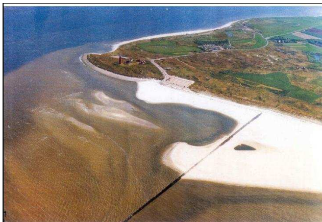
Figure 12.8 Long dam Texel
