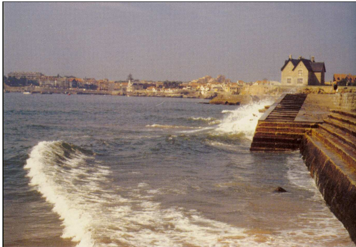
Figure 12.1 Seawall (Cascais, Portugal; high water, no beach in front of seawall)
