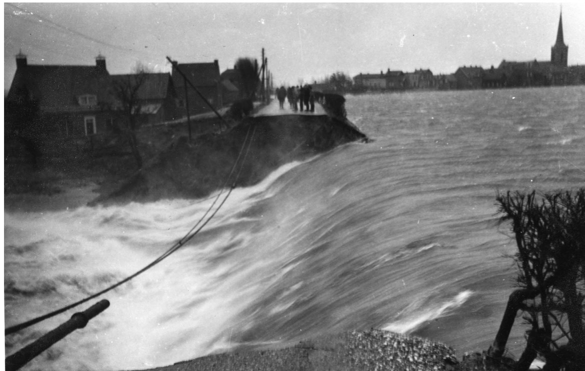
Figure 19 | A photo of one of the breaches of the flood in 1953 in Zeeland. You can see the speed that the water has when flowing to the hinterland, leaving a path of destruction. (Source: Rijkswaterstaat)
