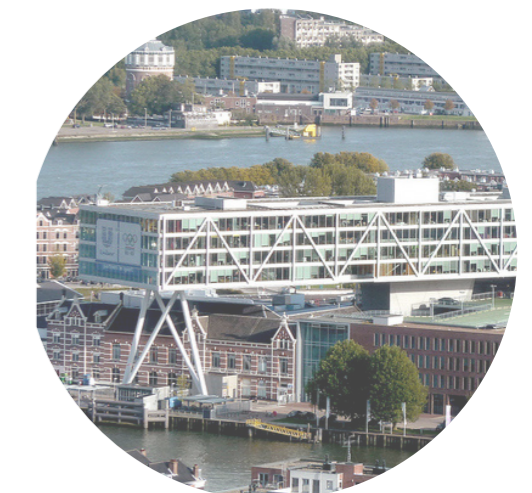
Figure 122 | Unilever Main office, design by JHK Architecten in collaboration with West 8, adds a building with external construction that goes over other buildings. (Source Image: Jan van Helleman)
