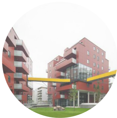
Figure 127 | Sonnewdviertel from Kada connects the semi public facilities like shared kitchen and laundry room with yellow hallways. With sharing these facilities the apartments can be smaller and therefore the building can accommodate more people. (Source: Kada)
