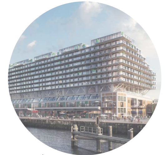
Figure 121 | Mei architecten designed an apartment building on top of the Phoenix food hall: the robust construction of the shed can carry extra load. (Source: Mei architecten)
