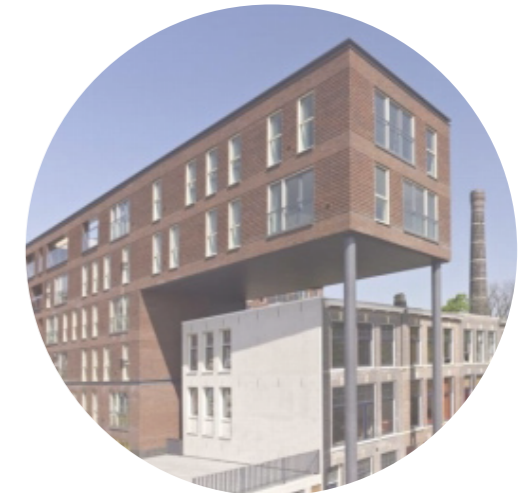
Figure 123 | Plegt-Vos made a construction over another dwelling building, without adding carry load to the old structure. The area can be densified in this way. (Source: Plegt-Vos BV)
