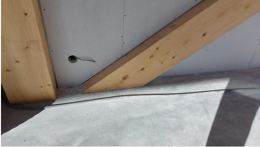
Figure 74: Wind brace in phase 2
