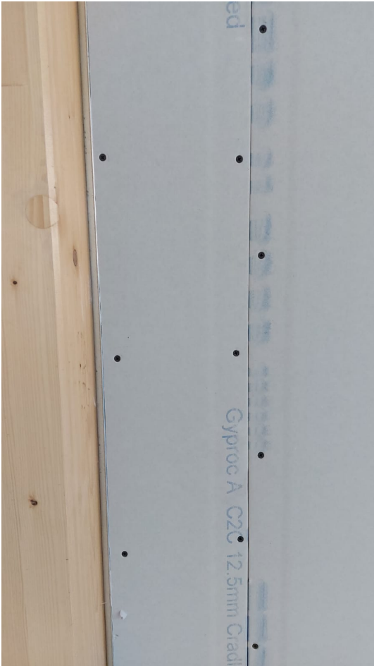
Figure 75: Connection column to partition in phase 2
