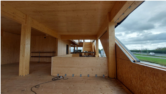
Figure 72: CLT floor connection to stair opening in phase 1
