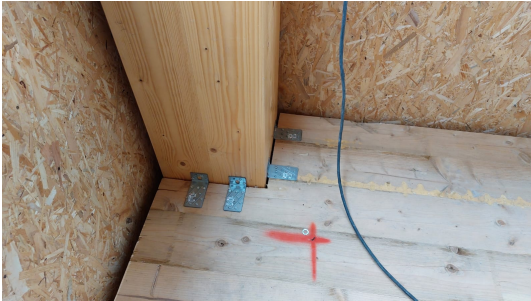
Figure 70: Corner column in phase 1
