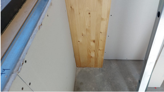
Figure 73: Corner column in phase 2
