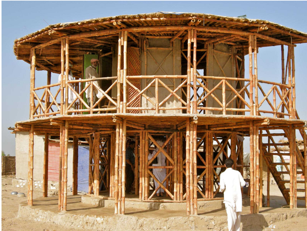
Figure 29: A bamboo shelter designed by Yasmeen Lari Heritage Foundation of Pakistan (2020)
