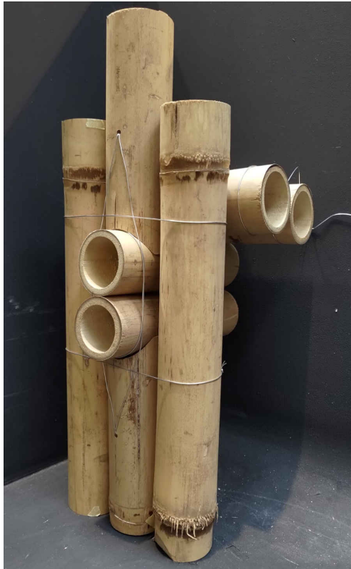
Figure 30: Modelling a bamboo joint that can be made without power tools by the local people themselves. This fragment was developed based on the techniques observed in the works of Yasmeen Lari. It is a fragment taken from a section from the left side of the detail section in Figure 23.
