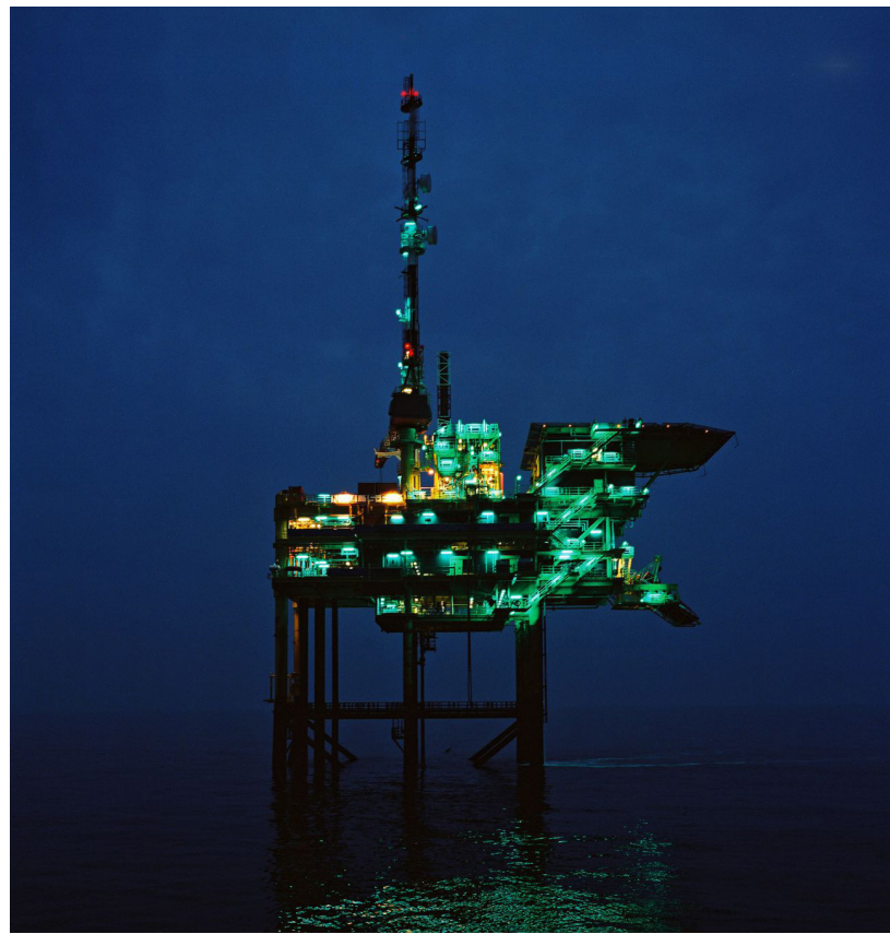
Figure 7.7: A drilling platform with green lighting to prevent disturbance of birds
