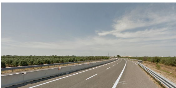
Primary Infrastructure A14
