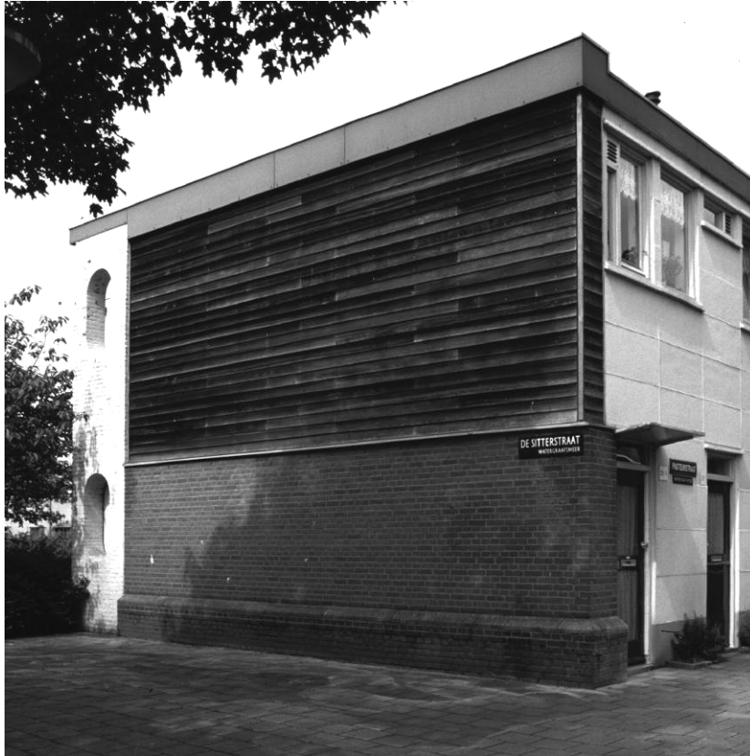
Figure 13: facade covered with wood and brick around 1987.
