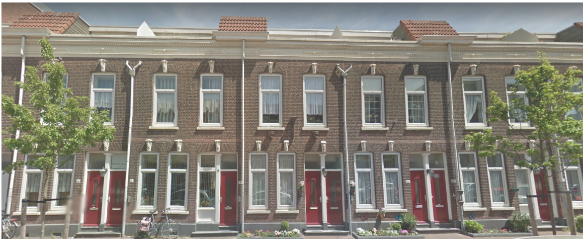
Figure 71 | In this street in Katendrecht personalized pavement is already happening. Small gardens and terraces make the street more lively. Also the door has small steps in front, that prevents the house from flooding (for a while) The steps could be made higher to increase this effect) (image by Google earth).
